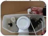
Reconnect the cable sheath carefully to the tank.
